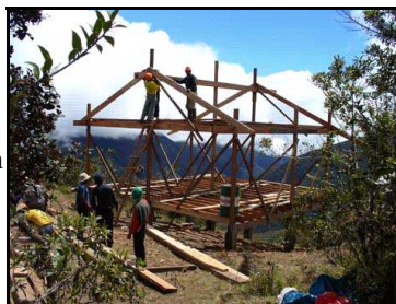
First cabin under construction at the Wayqechas Research Station
