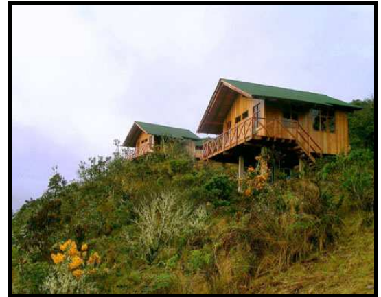
Wayqecha cabins overlooking the Kosñipata valley
